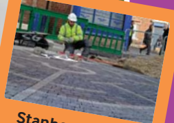
Stanhope Street - major revamp underway in the heart of Arthur's Hill
